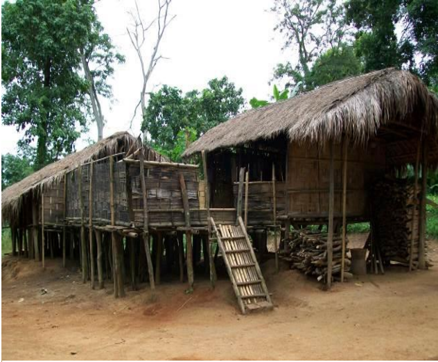
Fig. 2. Karbi traditional house constructed from bamboo
